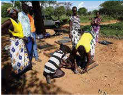
Women masons making toilet slabs - Katopoten village, Amudat district
