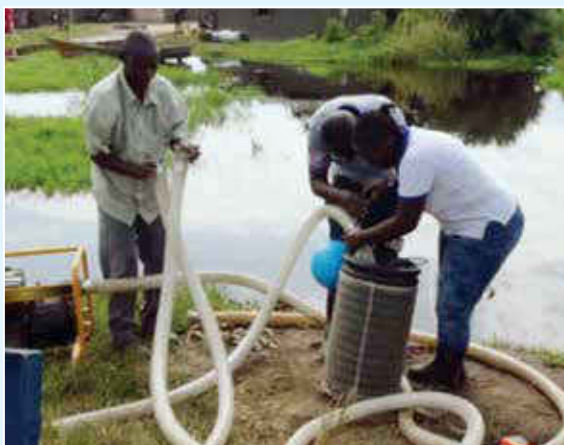
Photo 9- 14: setting up mobile water treatment
