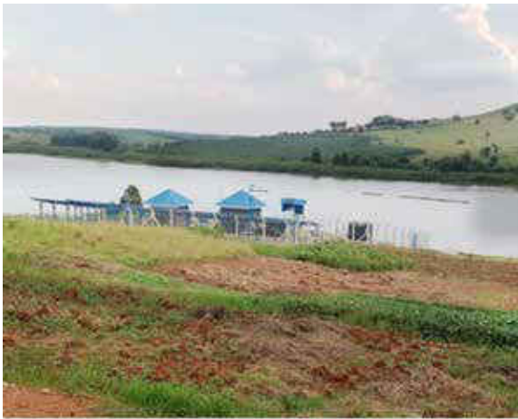
Photo 8-1 Mabira earth dam in Mbarara District
