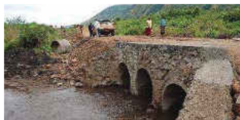
e) Kitebere landing site in Kagadi District at 80% physical progress
