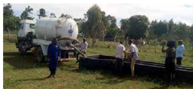
Photo 7- 7: Cesspool Truck emptying sludge at Kayunga FSTP
