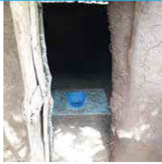
Completed latrine using pre-cast slabs embedded with sato pans - Katopoten
