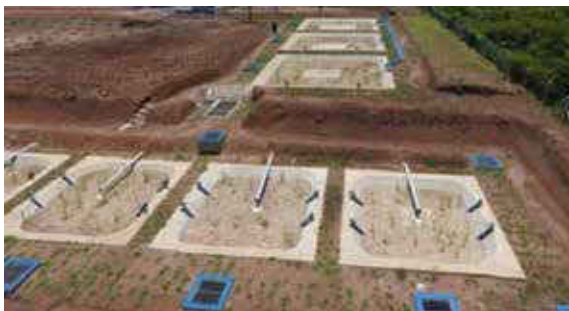
Photo 7- 2: Dzaipi FSTP (after construction).
