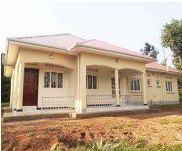
Photo 10- 22: Renovated staff quarters at Nyabyeya College
