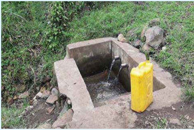
Photo12- 1: Kibande spring before GFS construction
