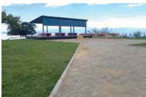
b) Mahyoro landing site in Kitagwenda District completed and politically commissioned by the Minister of State for Fisheries under Industry and
