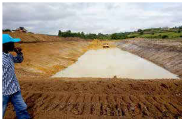
Photo 10- 10 Water retention facility for recovery Wetland in Sheema
