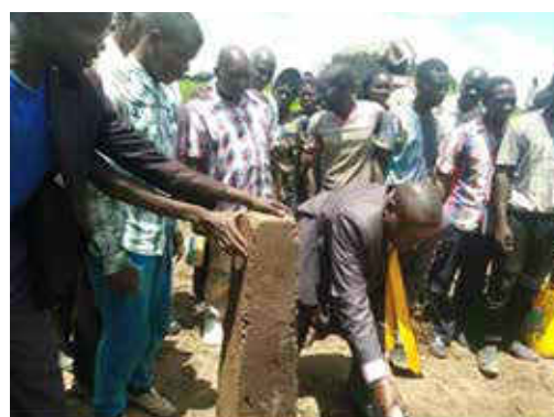
Photo 10- 6 RDC Soroti planting the first concrete pillar at Opiyai Wetland boundary, Soroti
