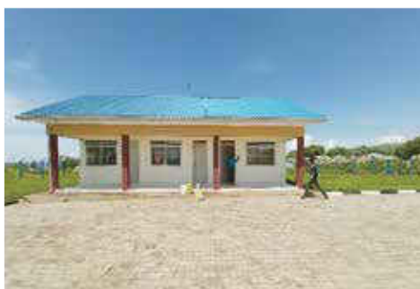
c) Dei landing site in Pakwach District at 97% physical progress
