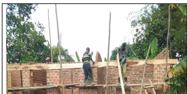
Figure 1 Construction of Staff quarters
