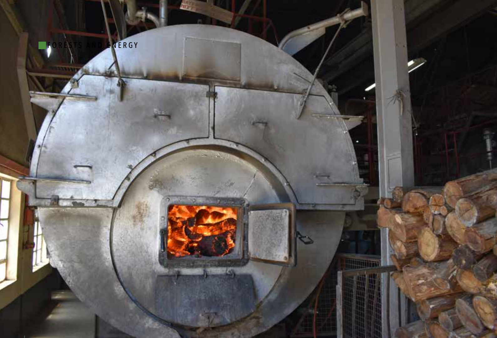
One of the furnaces at Unilever in Mufindi. Eucalyptus firewood on the right
