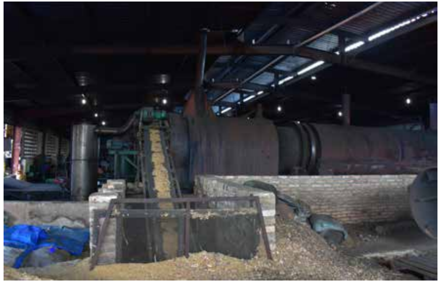
View of the conveyor belt that feeds the furnace with wood particles & waste
