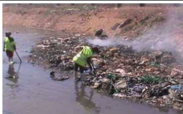
Figure 2. KCCA workers cleaning of Nakivbo Drainage Channel. Photo by Environmental Alert.
