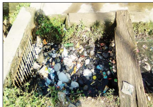
Figure 2: Indiscriminate waste disposal in drainage channel in Kiroombe Village, Makindye 1 Parish, Makindye Division, Kampala. Photo by Environmental Alert.
