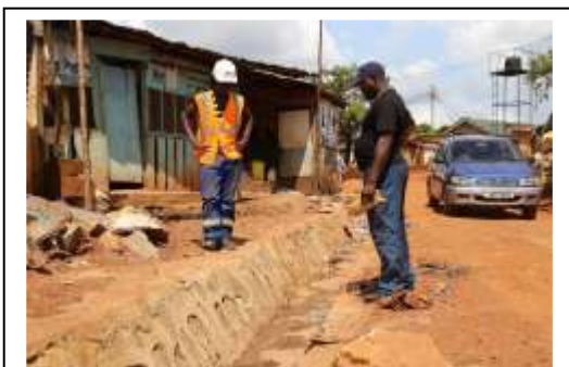
Figure 2: Francis inspects the lined section of the drainage channel accompanied by an Engineer of SOGEA SATOM. . Photo by Environmental Alert.
