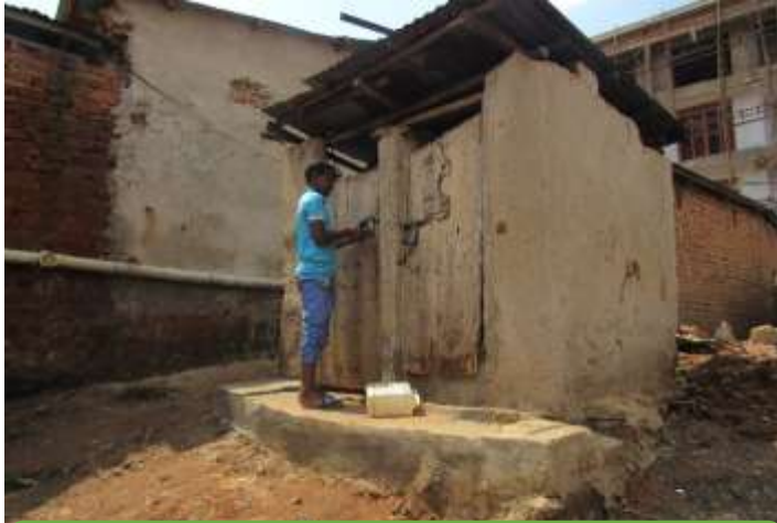
Figure 1: A student of Madarasa School accesses the toilet facility
