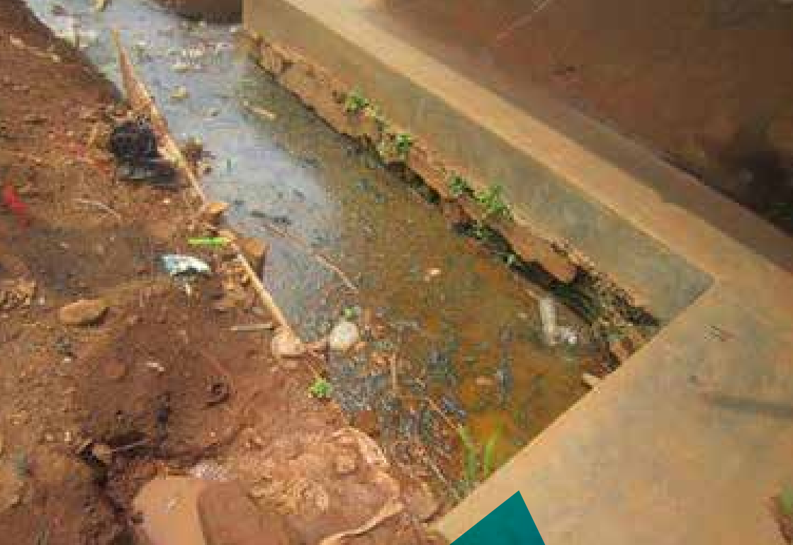
Figure 12: Unlined drainage with stagnant water, silt and disposed solid waste in Bulagani zone, Baise III Parish in Kawempe Division.
