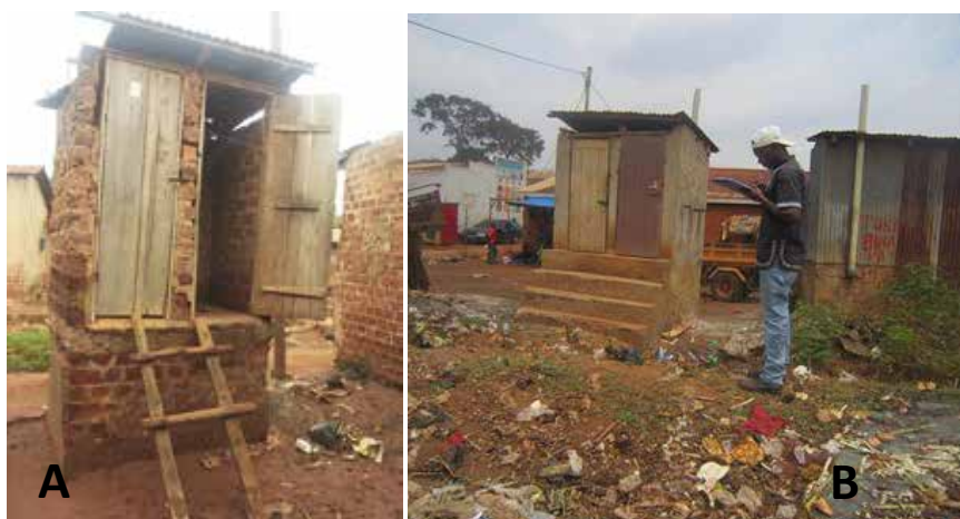
Figure 11: A simple pit latrine and B is Pit latrine with a vent pipe in Kisenyi zone, Bwaise I Parish in Kawempe Division .
