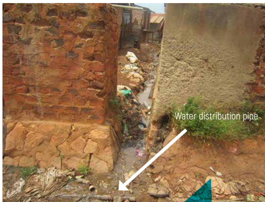
Figure 23: Water distribution line passing via unhygienic drain in Kifumbira zone, Mulago III Parish in Kawempe division.
