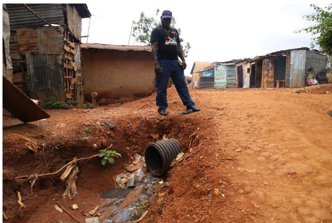
Figure 3: Francis inspects the new pipe that SOGEA SATOM put in place of the old broken culverts.
