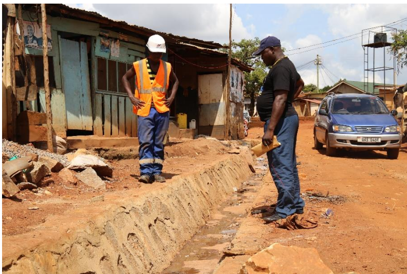
Figure 2: Francis, a VHT of Mbuya II ward inspects the lined section of the drainage channel accompanied by an Engineer of SOGEA SATOM
