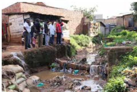
Figure 15: Solid waste dumped in a drainage channel in Mengo ward.
