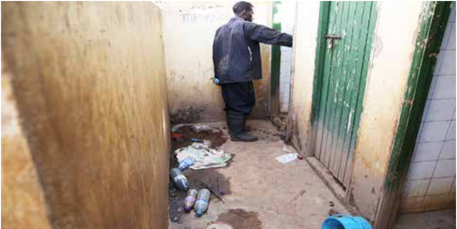
Figure 10: Poorly maintained public Toilet in Bukesa ward, Kampala Central Division.
